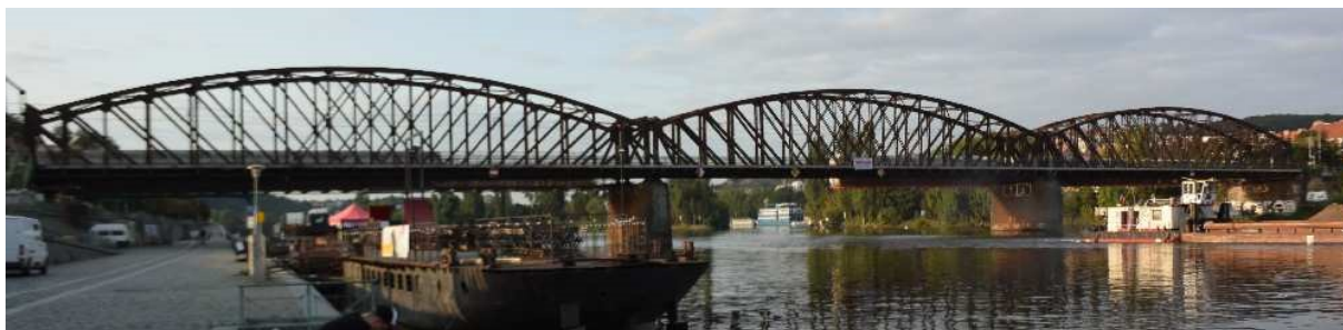
Fig. 1: View of the railway bridge under Vyšehrad
