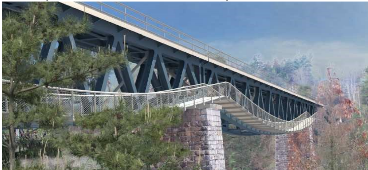
Fig. 14: Visualization of the bridge with a footbridge
