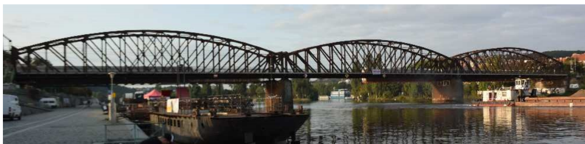
Fig. 1: View of the railway bridge Pod Vyšehradem
