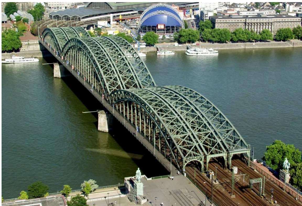
Fig. 16: Aerial view of the bridge
