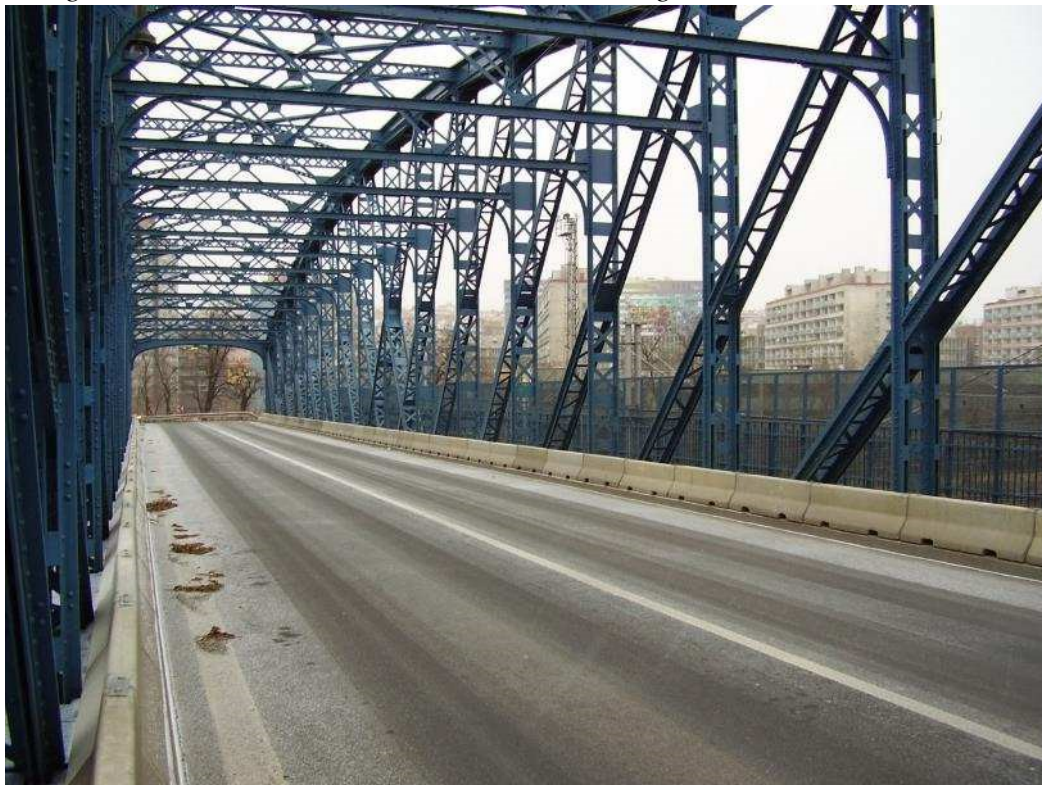
Fig. 4: Partial view of the bridge construction
