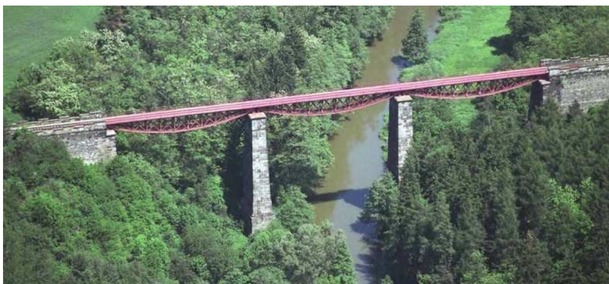
Fig. 6: Aerial view of the bridge
