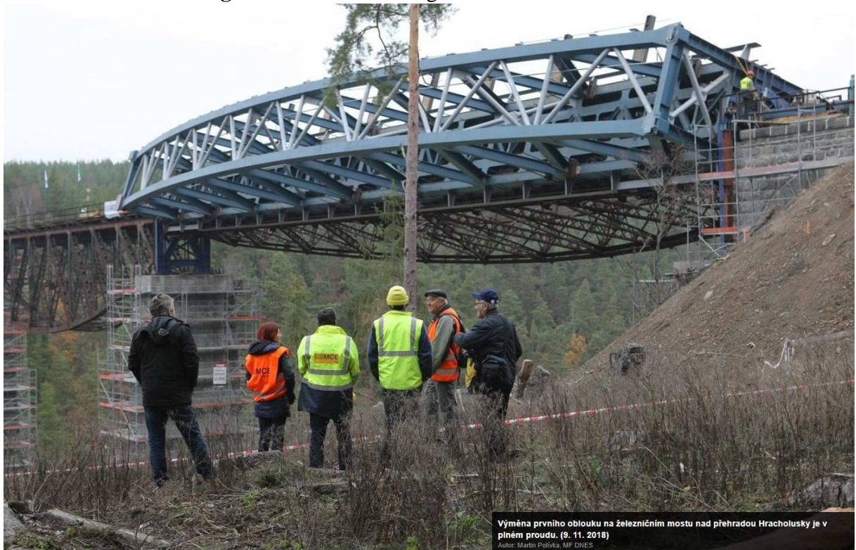
Fig. 13: Replacing the first arch
