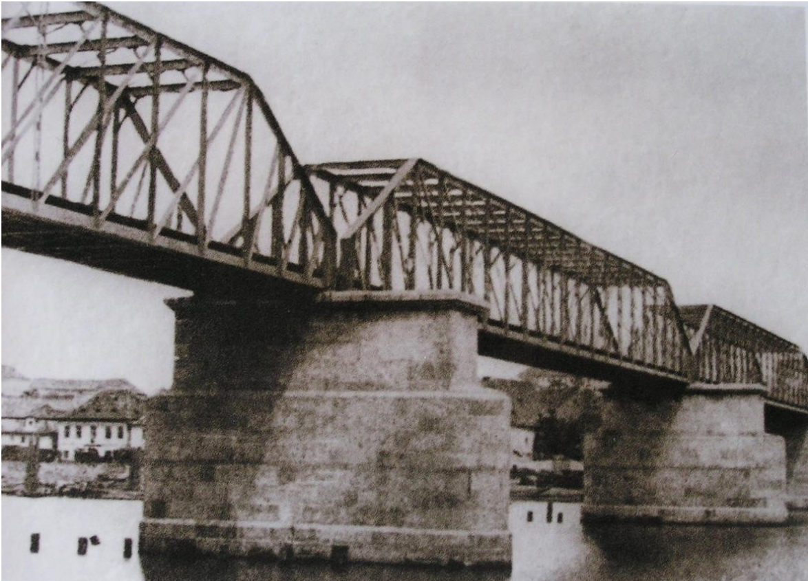
Vltava River bridge from 1874 (photo by F. Fridrich)
