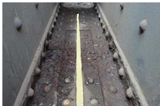
TYPICAL CORROSION OF THE LOWER CHORD IN THE SECTION BETWEEN THE PANEL POINTS
