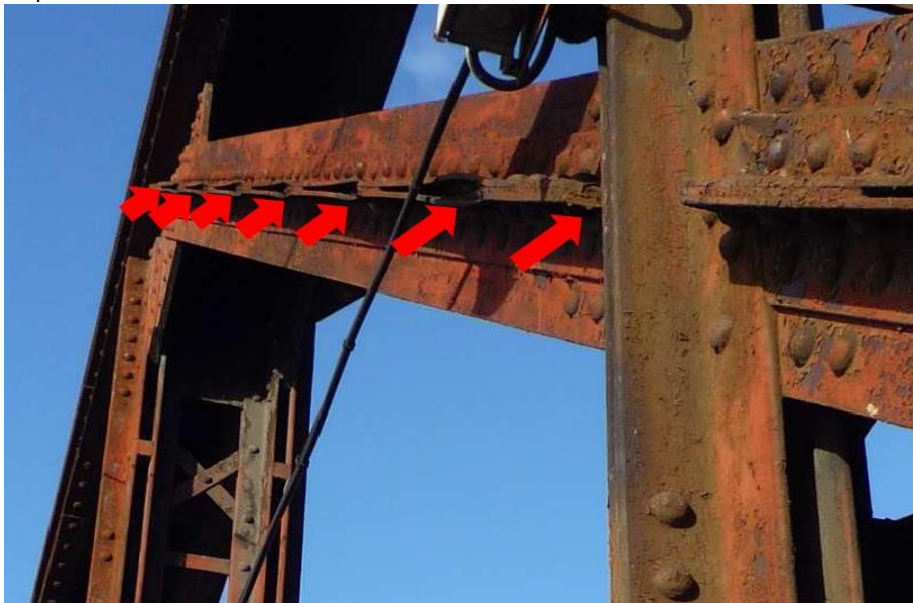
Severe crevice corrosion in the connections of the couplings of the segmented rods of perpendiculars and lacings
