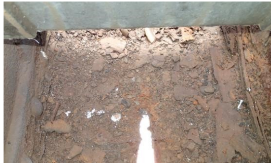
TYPICAL CORROSION OF THE LOWER CHORD IN THE SECTION BETWEEN THE PANEL POINTS
