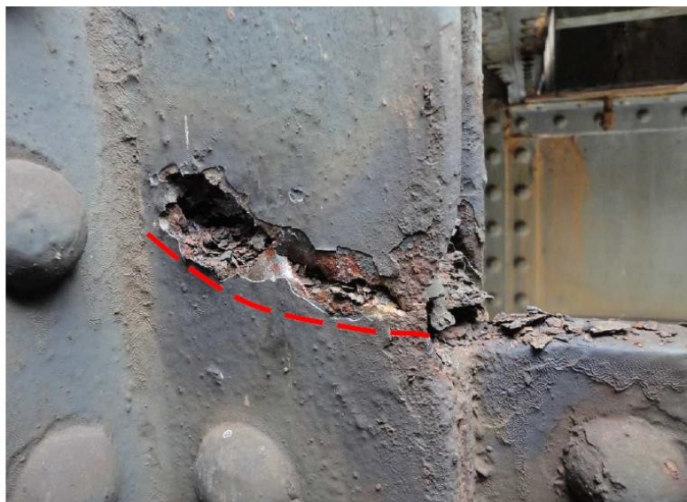
Corrosion in the connections of perpendiculars and lacings to the splice plates of the lower chord
