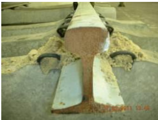
Fastening System covered with sand
