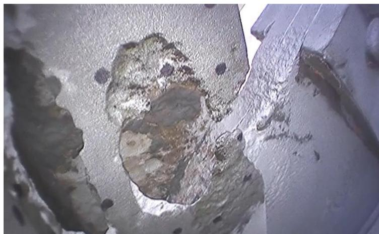
*Photo source: video by Faculty of Civil Engineering, CTU, corrosion captured by endoscopic probe on the diagonals of the Výtoň bridge, September 2023*
